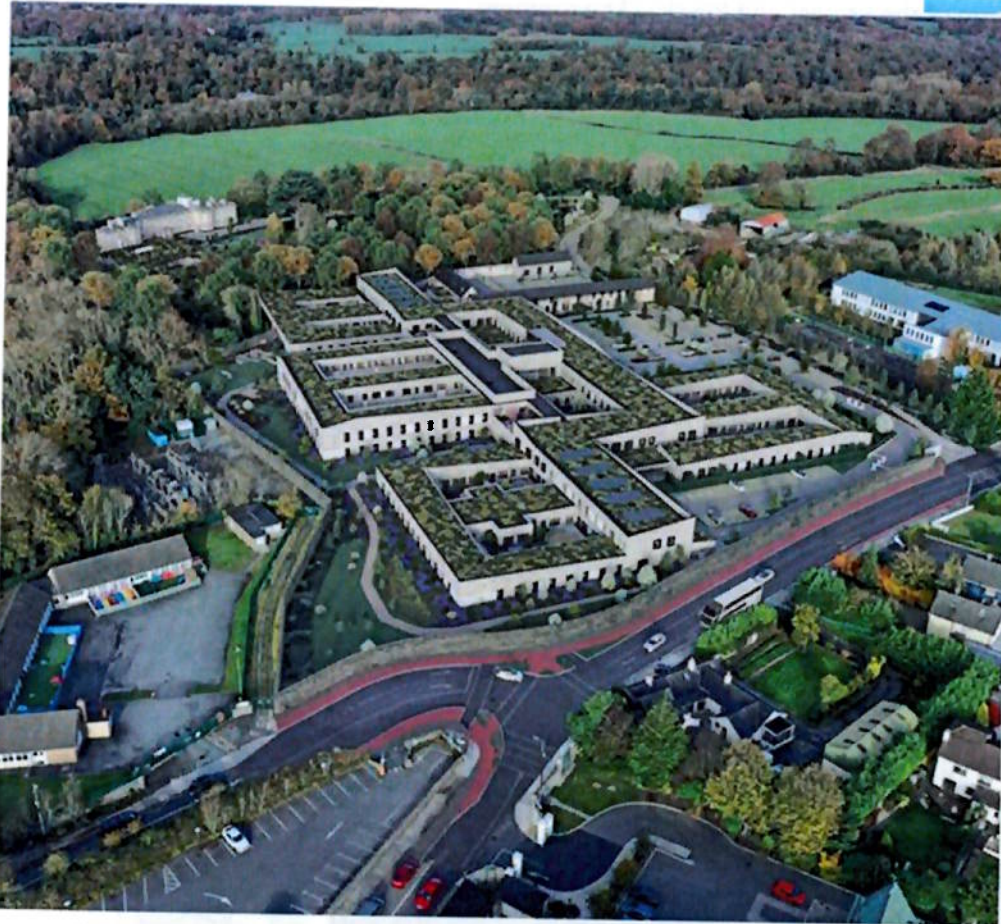
Figure 1-3: Aerial View of the Proposed Development
